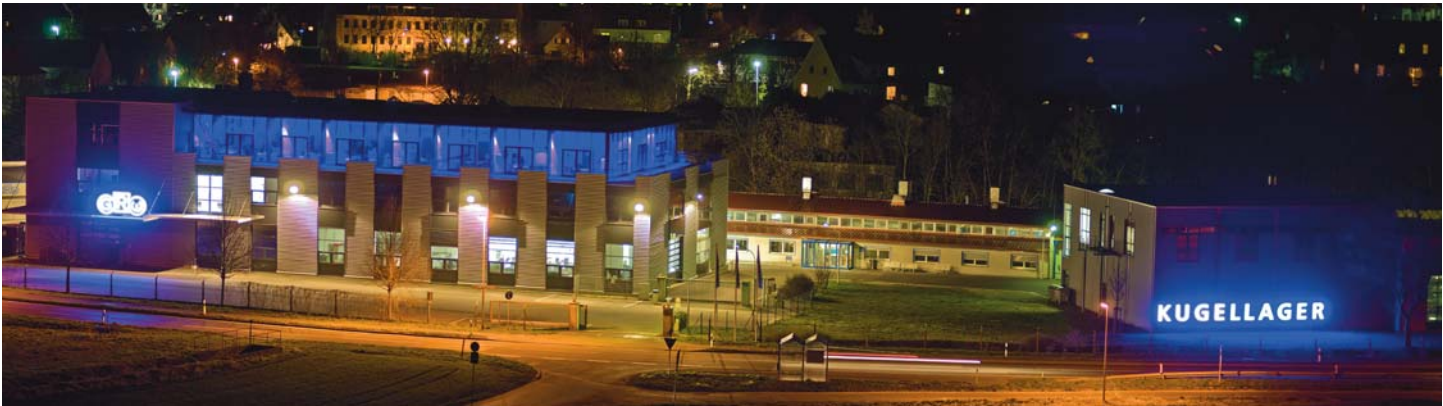
Headquarter and production site at Rimpar
